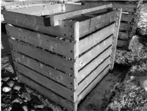
Photo 1. The completed compost bin showing the removable slats held within a slot formed by two upright 2x2's. The cross bar prevents the sides from bowing out when the bin is being filled. In this case the bin is sited on concrete pavers and the lower portion of the 2x2's were sawn off to leave a 1 inch space beneath the lowermost row of planks
