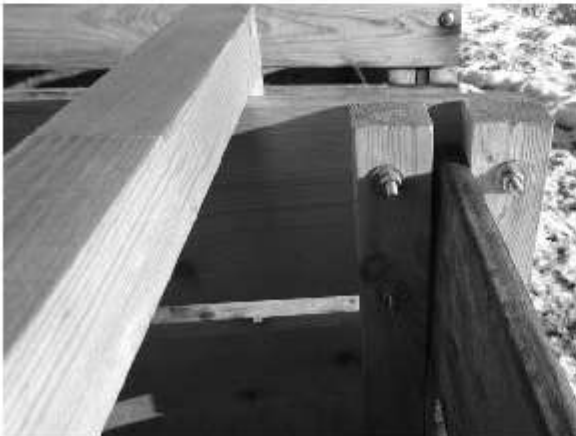
Photo 6. Detail of slot for the removable slats. Note that the inner post that forms the slot is held in place only by two bolts at top and bottom. The crossbar is seen in its proper location towards the front of the bin.
