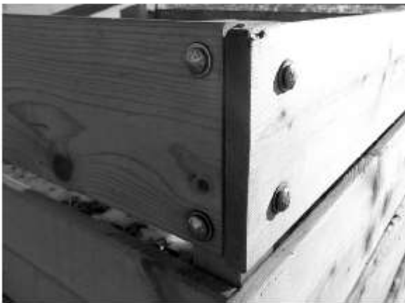
Photo 2. Upper back corner showing the side plank that overlaps the back plank. The photo shows the offset of the bolts that allows the bolts to pass through the 2x2 without interference.. Also visible is the cupping of the plank. Care has to be taken not to overtighten the bolts during assembly to prevent splitting the plank.
