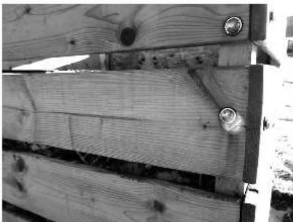
Photo 3. The centre planks below those of Photo 2. The centre boards are only attached by a single bolt. The bolt on the side plank (right) is centred but the one on the back plank (left) is offset upwards; again to allow clearance of the two bolts as they pass through the 2x2.
