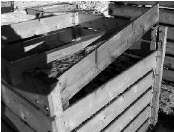
Photo 5. shows a slat partly removed and resting on its spacer. Behind it is the crossbar.
